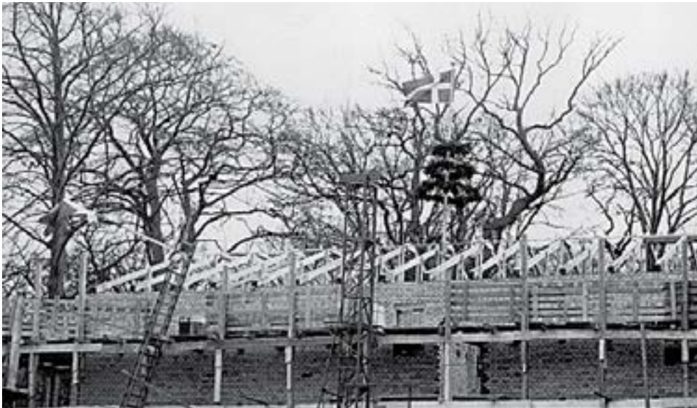
Ceremony for raising the roof-tree at DBL’s premises.
