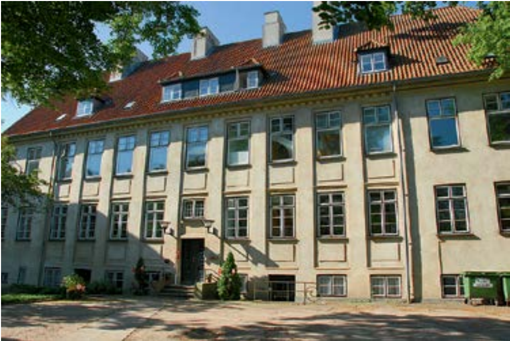
The building at the Frederiksberg campus, KU, where DBL was hosted from 2008.
